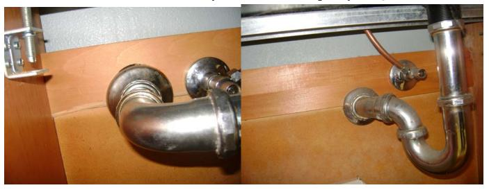
Drain piping and supply tubing for the sinks were sealed through the engineered wood panels that formed the back of the science classroom cabinets; however the panels were separated from the wall by a two inch gap.
