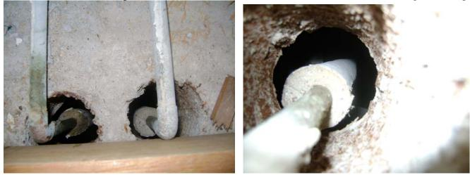
Tubing came through unsealed floor penetrations from the sub-floor space. Holes were large enough to allow animals and moisture laden air to get behind cabinetry to leave feces droppings and create mold development.
