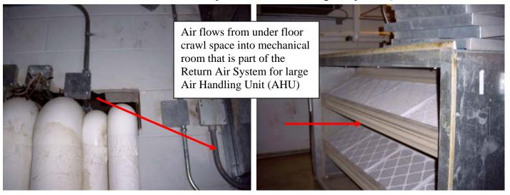
Unsealed piping penetrations through an under ground exterior wall allowed contaminated air to be suctioned into the Return Air Stream of a multi-zone air handling unit that supplied air to an entire wing of a school.
