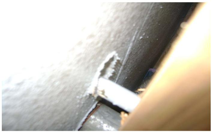
The two inch gap between the back of the cabinet panels and the sheetrock wall allowed air to flow through the unsealed pipe penetrations in the sheetrock. Moisture laden air was getting into the back of the cabinets and fostering mold development in the drawers and on the surfaces of the engineered wood panels.
